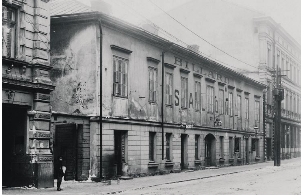
In the early 1900s a billiard saloon stood where the Helsinki Stock Exchange building would later be raised.
